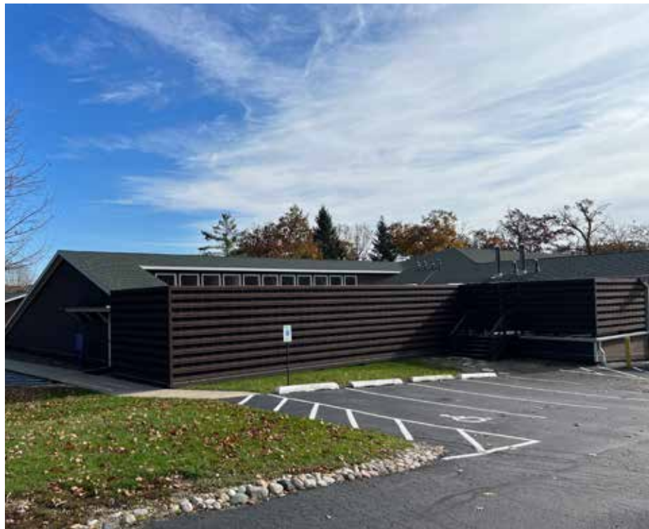
Existing dining facility and kitchen
