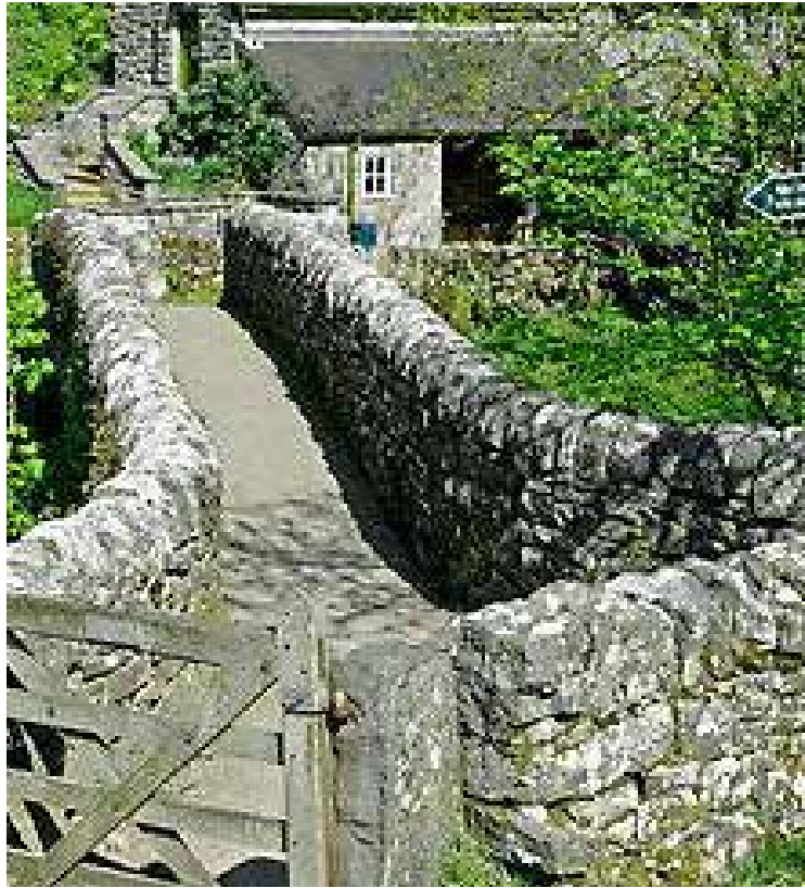
Stone Wall Cabin Garden
